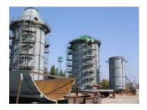
The size of the 4 radiant modules range from 4.5 m diameter by 10 m high to 8.6 m diameter by 18m high will be shipped in a full module with approx total 340 tonnes for four units.
