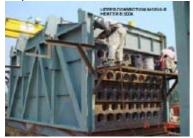
Each of the heaters' radiant sections were completely assembled at the Unithai's factory prior to delivery with radiant coils (2no. of SS321 stainless steel and 3no. of A-106 carbon steel) and internal ceramic fiber lining installed.
