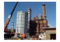
Steel Tonnage 145 tonnes Shipping Weight 335 tonnes Coil Materials P5 Owner Caltex Employer Foster Wheeler Location Australia Completion Date January 2003
