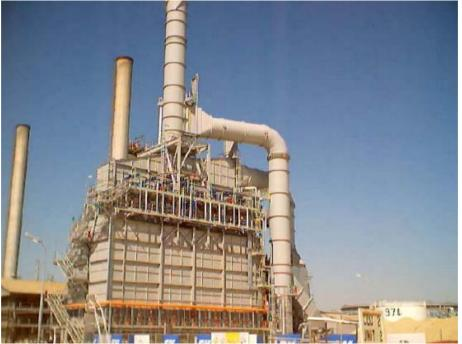
As part of Kuwait National Petroleum Company's (KNPC) on-going development plans for its Mina AI Ahmadi refinery, ABB Lummus Heat Transfer (LHT) was called on to design and install a new crude heater, to replace the existing Crude Distillation unit known as CDU#3
