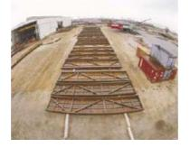
Unithai's scope of works covered the fabrication of radiant section steelwork for a pair atmospheric and a pair vacuum column feed heaters. Each pair of heaters shared a common stack.
